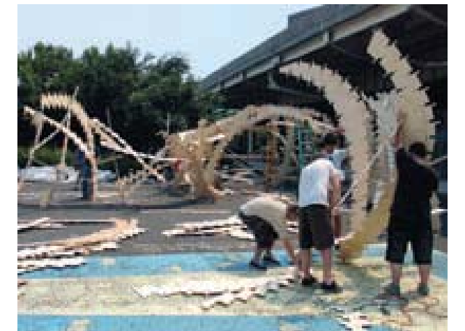
Deploying the pavilion at the CitySol Festival. Solar Pavilion 2, SITU Studio, 2007, Photo courtesy SITU Studio
