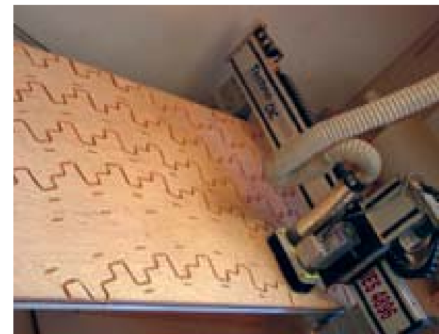
CNC router cutting .5 in. plywood sheet. Solar Pavilion 2, SITU Studio, 2007, Photo courtesy SITU Studio
